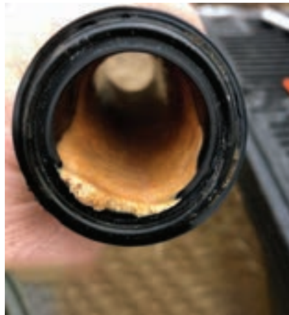
Mats of bacterial biofilm in a stainless steel dairy pipe.
